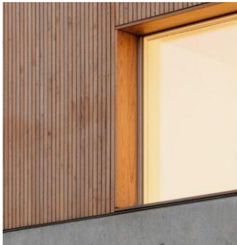
Vertical timber look cladding and timber window reveals
