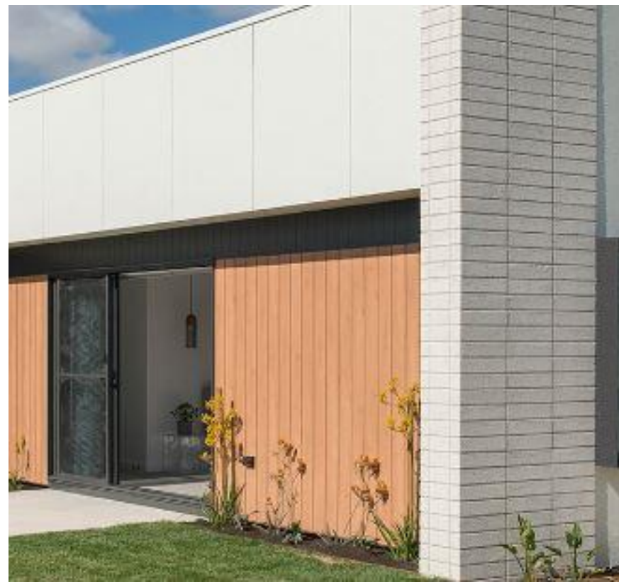
Combination of face brick and vertical caldding
